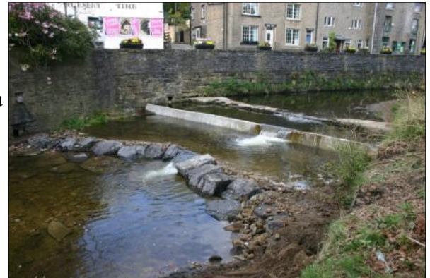
Step system at weir two.
