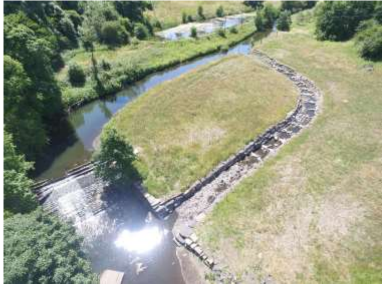
Figure 4.1. Oakenshaw weir and bypass channel Summer 2017 before 1.2ha of woodland planting took place in the winter.
