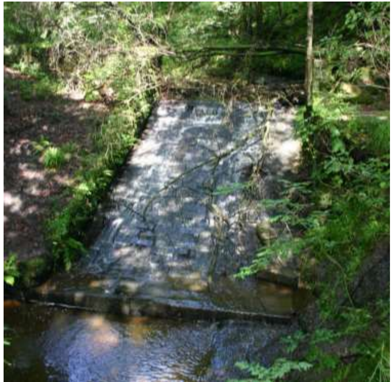
Figure 3.9. Duddel Brook weir on the Lower Ribble August 2018.
