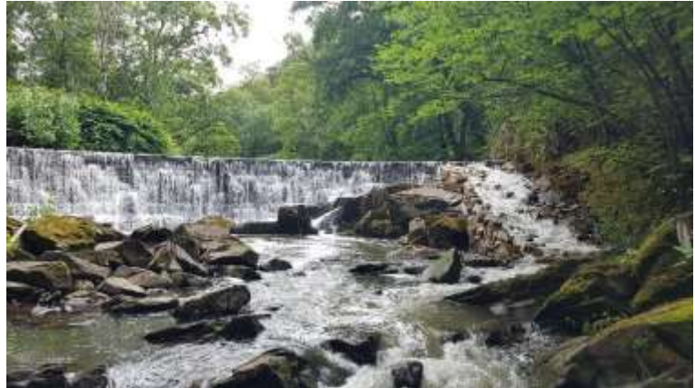
Figure 4.2. Hoghton Bottoms Weir and fish pass. Summer 2018
