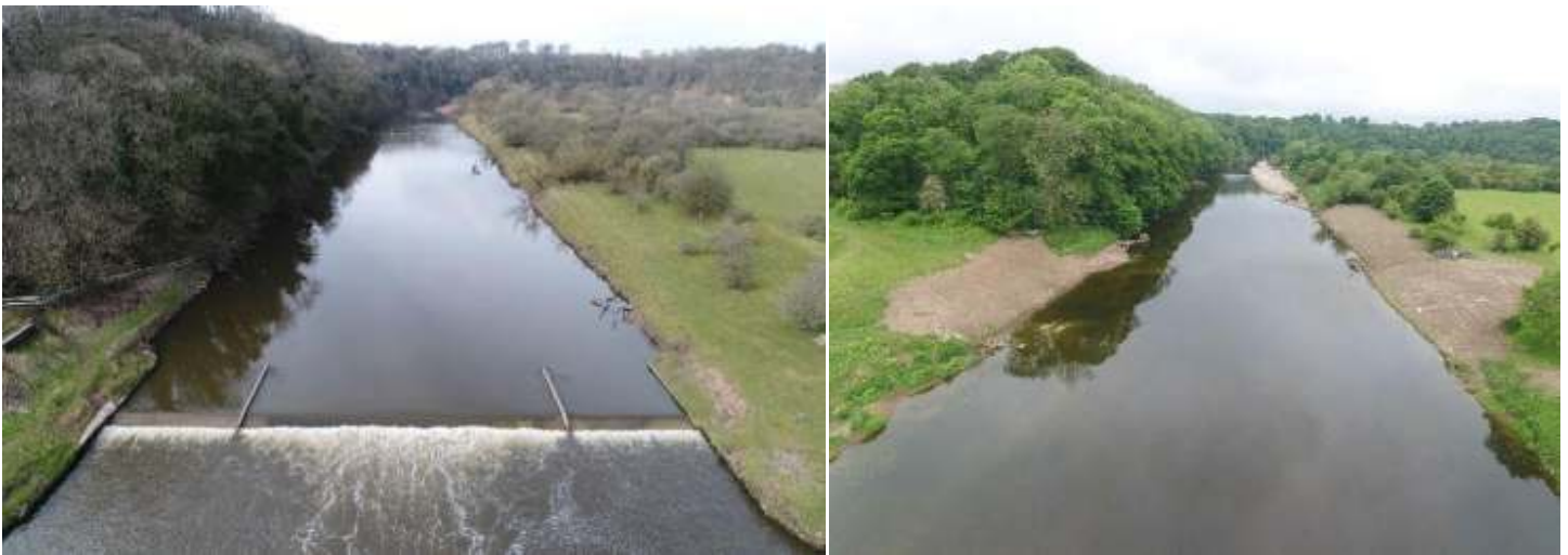
Figure 4.0.5. Samlesbury Weir removal on the River Ribble, Samlesbury. Today, the widest weir removal in England
