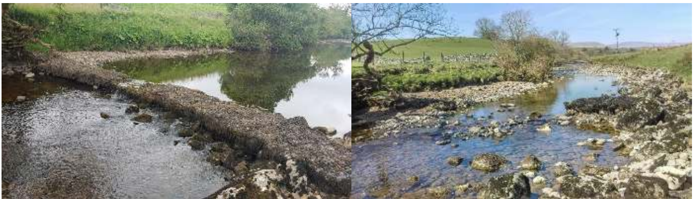
Figure 4.0.4. Partial weir removal on the river Ribble in the Upper Ribble near Horton-in-Ribblesdale
