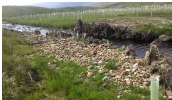
Figure 4.0.1: Berm features installed by Ribble Rivers Trust - Gayle Beck 2020
