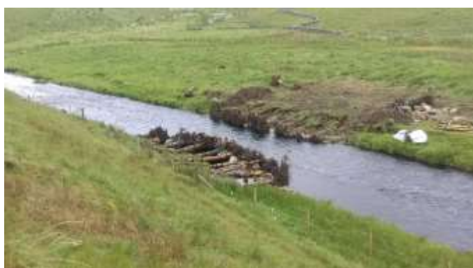
Figure 4.0.1: Berm features installed by Ribble Rivers Trust - Gayle Beck 2020
