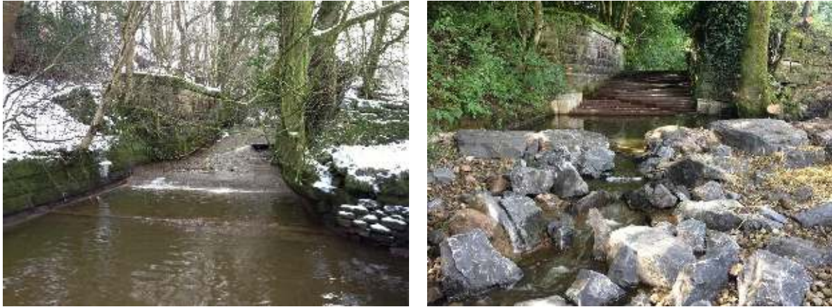
Figure 9 Photo's above show a fish easement solution of a previously impassable weir on the River Loud before (left) and after (right).
