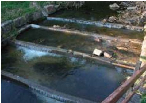
The River Don weir after
