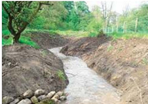
Ings Beck with the off-stream spawning channel in place
