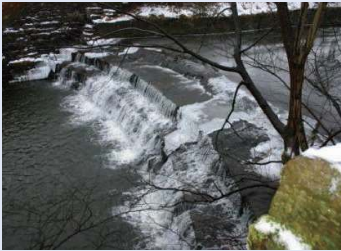
A weir at Barrowford Weir before fish pass construction
