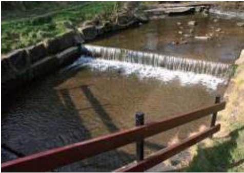
The River Don weir before
