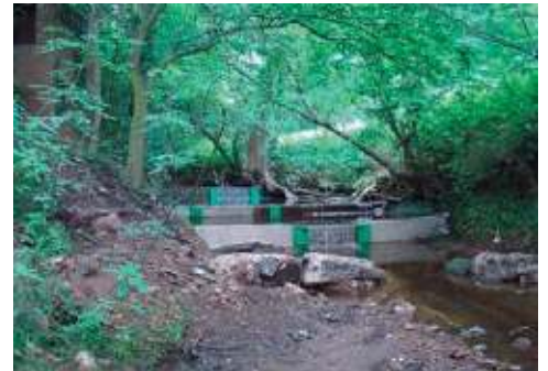
Bezza Brook weir after
