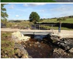
The next step was to tackle an old concrete ford that was partially obstructing the path of migratory fish. The existing structure was removed completely and replaced with a new bridge, complete with removable rails to allow for wider farm machinery. The channel sides were reinforced with boulders, which were donated in kind by Hanson Cement.
