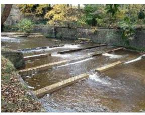
weir on the River Brun in Thompson Park drew additional funding from the River Improvement Fund. The construction of the fish easement was challenging as wet weather and subsequent high flows caused long delays. However, the finished design works well and it is another step closer to opening up the River Brun to migratory fish.
