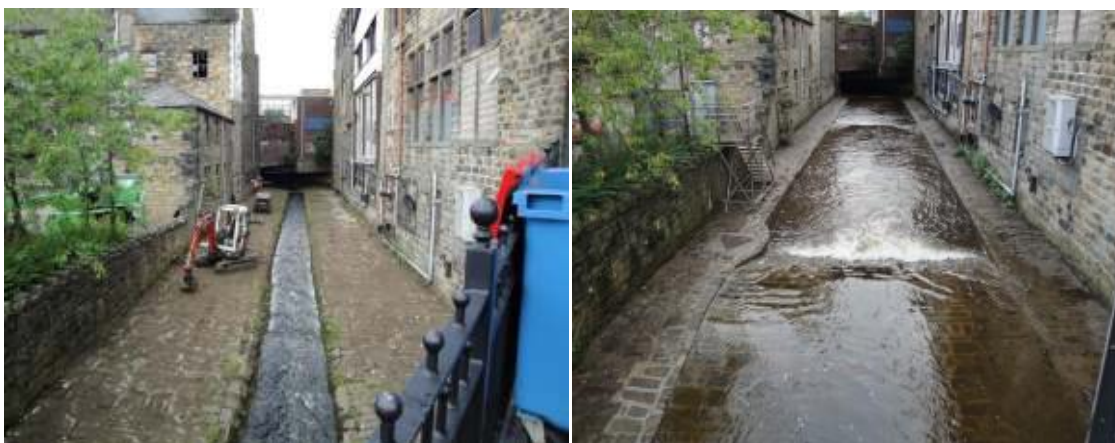
Figure 3 – Site 9 before (left) and after restoration (right)
