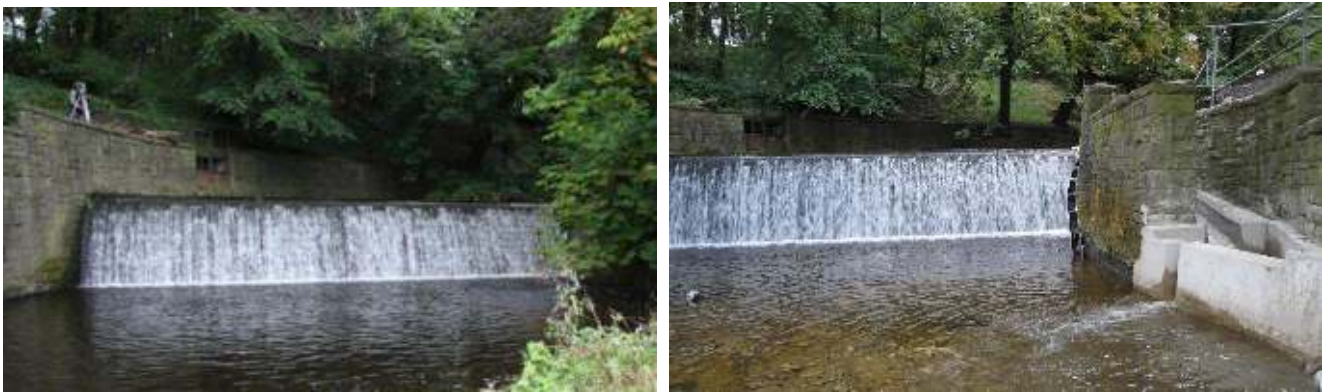
Burnley Weir before and after fish pass installation
