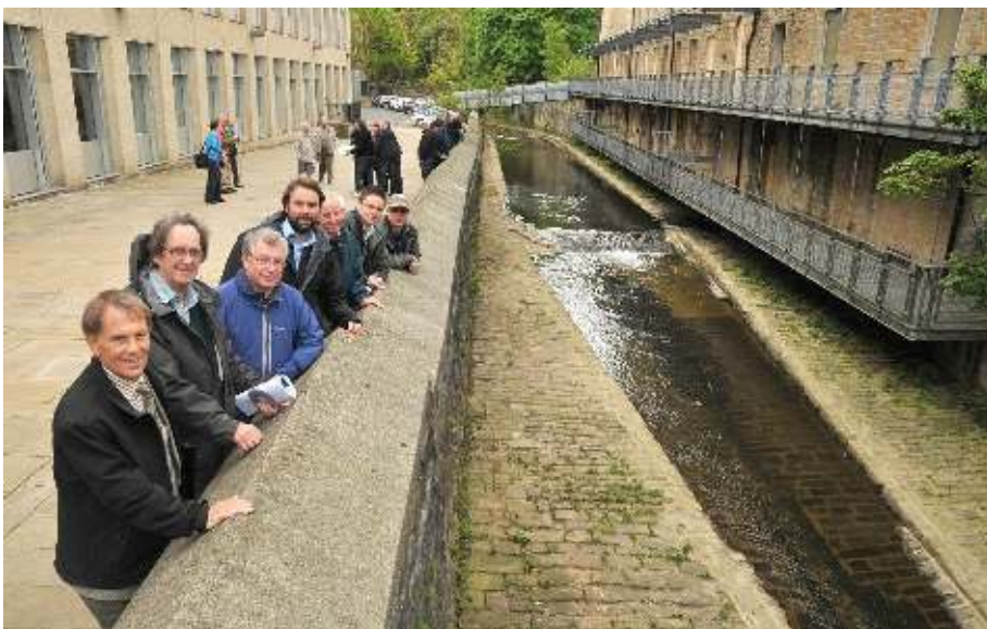
Members of the steering group visit the completed works at Calder Reach 5
