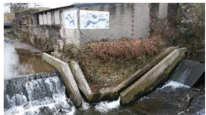
Confluence of the Rivers Brun and Calder today, featuring fish passes that allow migrating fish access upstream for the first time in decades. Furnished with artistic interpretation panels.
