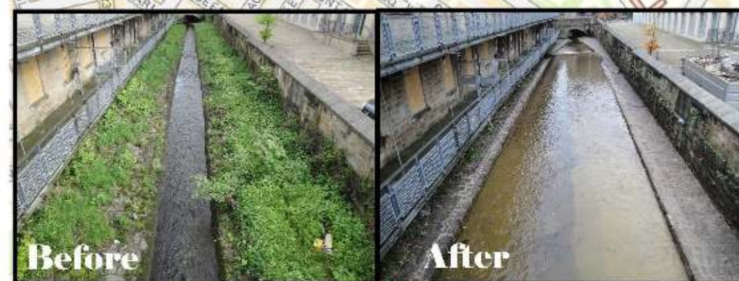
River channel improvements
