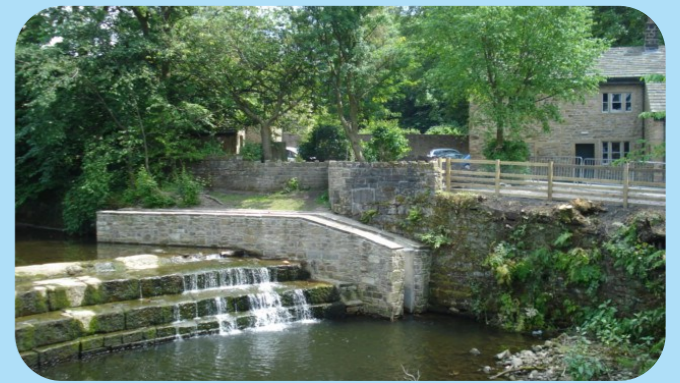
The completed fish pass in July 2011 including viewing platform next to Pendle Heritage Centre.
