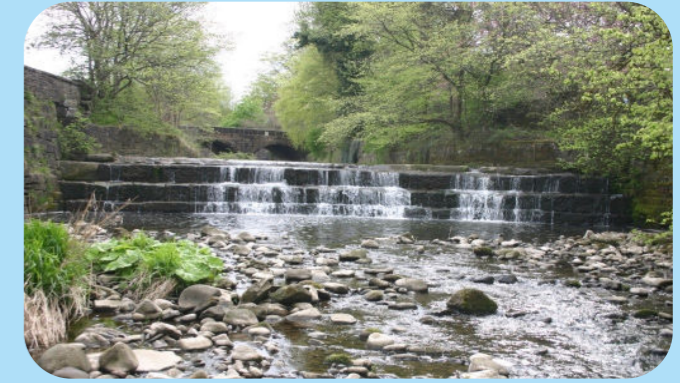
Barrowford weir before alterations.
