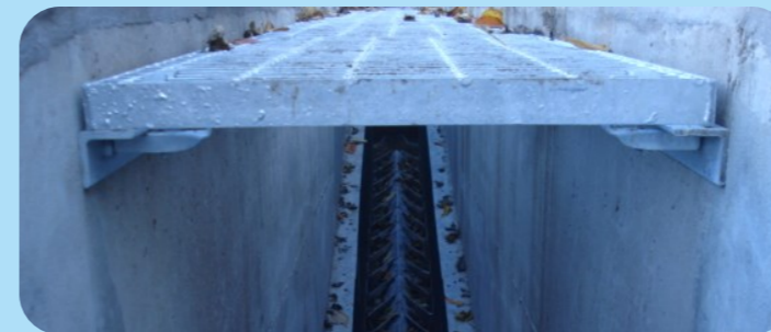
Baffles inside the fish pass during construction.
