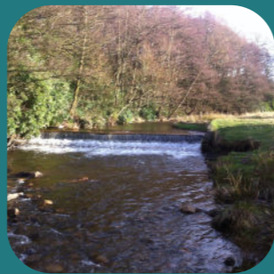
Before: The weir formed a barrier to fish migration.
