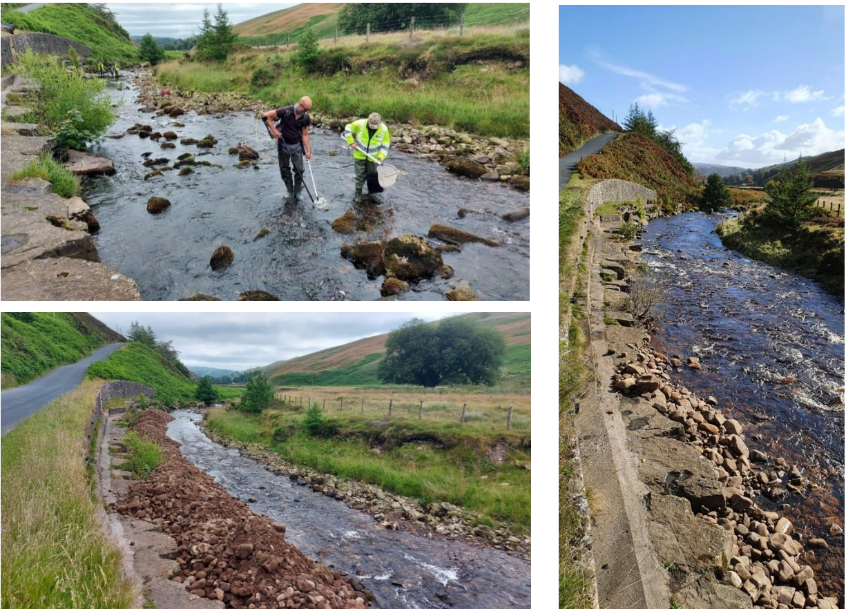
Figure 4.2.1: Ribble Trust and EA electric fishing teams catching and relocating fish on Langden Brook before gravel introduction (top left); gravels introduced along bank for redistribution in high flow events (bottom left); remaining gravels after first October high flow event (right).
