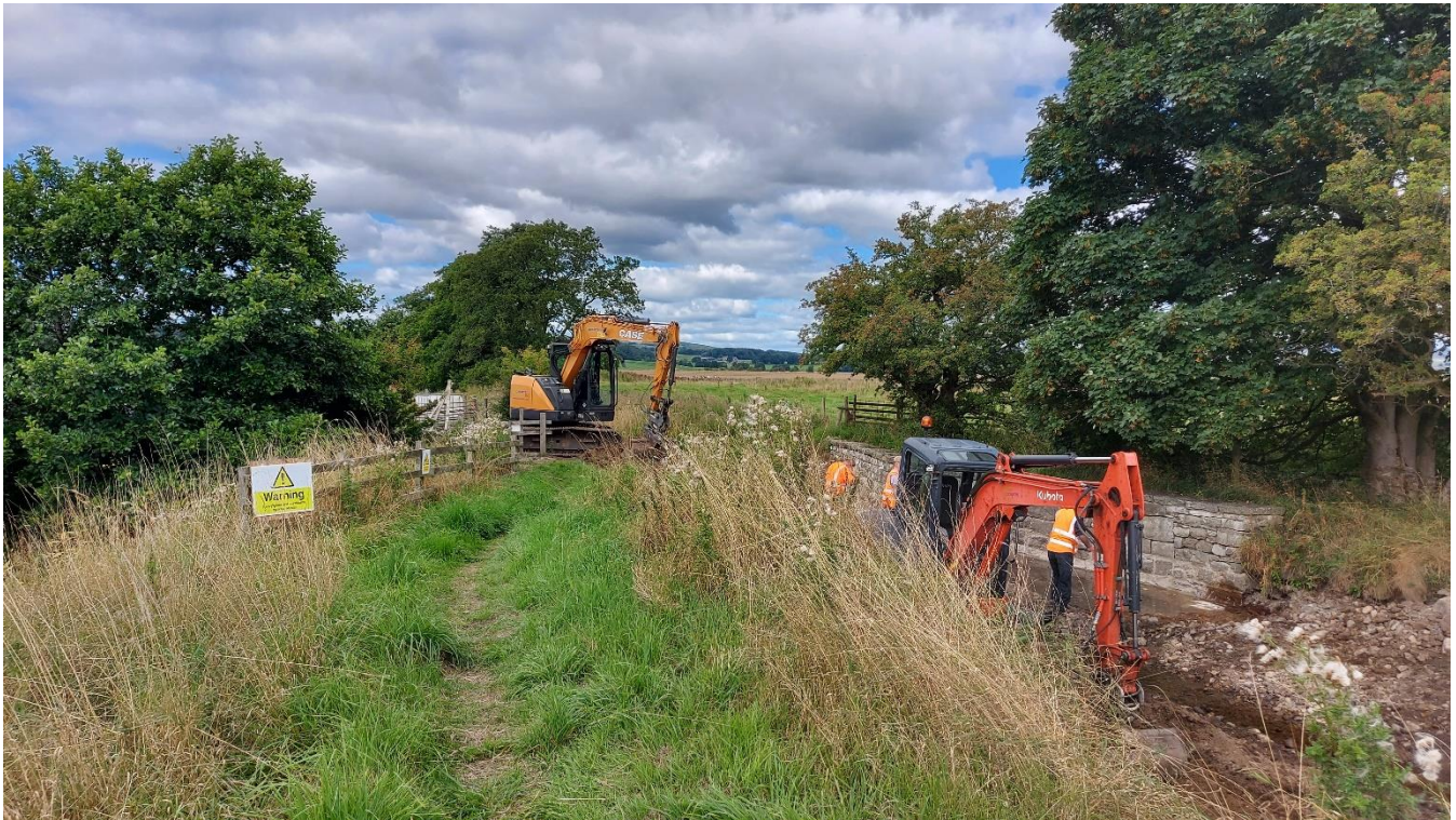
Figure 4.4.1: Wigglesworth Beck aqueduct repairs summer 2022.
