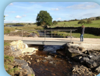
After: Bridge over Easington Brook
