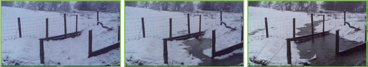
Images above: timelapse photos show the off-take channel in operation in a large storm event in February 2020.
