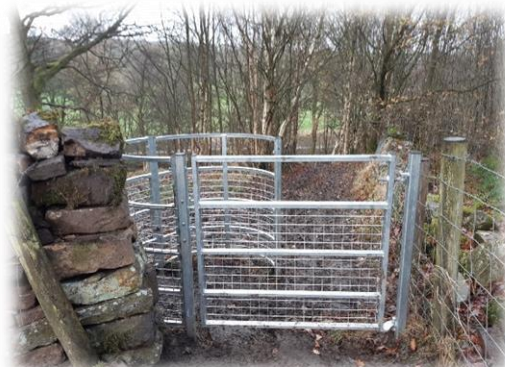
After: kissing gate installed at Wet Marl Wood, Burnley
