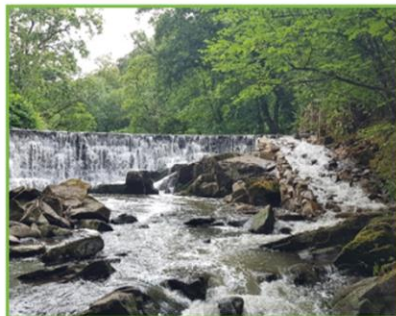
Image left: Hoghton Bottoms weir pre- and post-construction of fish pass.
