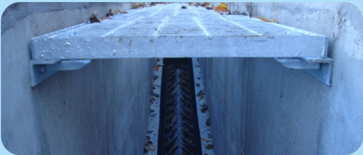
Baffles inside the fish pass during construction.
